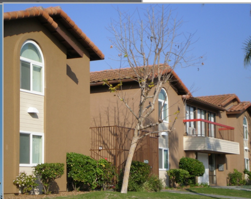
Alabama Manor, San Diego, CA / Community Housing Works Within 2 blocks of 4 major transit lines
