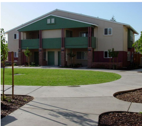
Mutual Housing at Norwood, Sacramento
